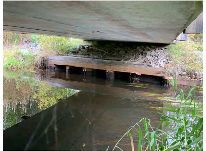
Left Bank Abutment when facing downstream
