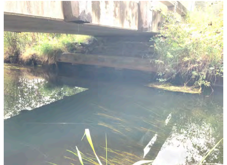
Right Bank Abutment when facing downstream
